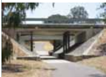
Bicycle (and pedestrian) underpass with clear sight lines; Canberra, Australia.
