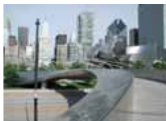
Pedestrian overpass; Millennium Park, Chicago (U.S.). Note, the metal railings do cut off views so the park is fairly heavily staffed with security.
