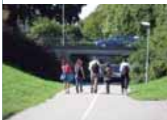
Underpass that is only partially below grade below raised roadway; Vallingby, Sweden. Sight lines are adequate.
