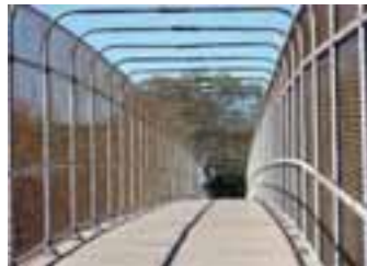
Bicycle and pedestrian bridge with adequate but uninspired design and curvature that limits sight lines; Minneapolis, (U.S.).
